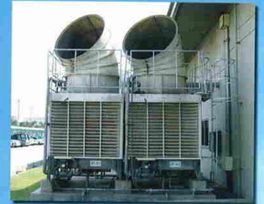
Closed circuit type (MXC)
