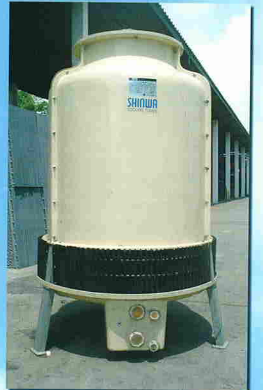
Counter flow type (SBC)
