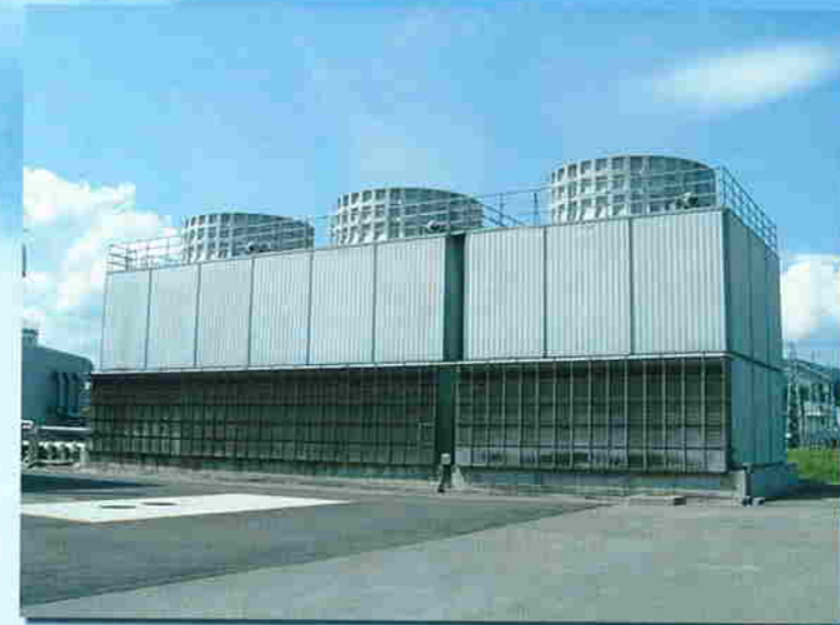
Counter flow type (SCC)
